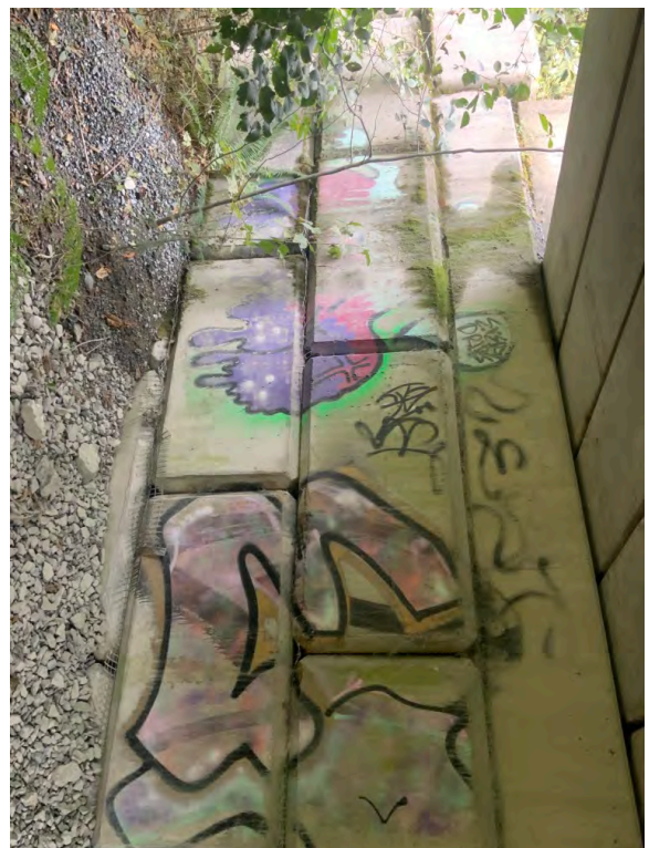
Right Bank Abutment when facing downstream
