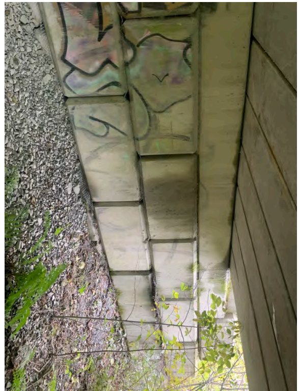
Right Bank Abutment when facing downstream
